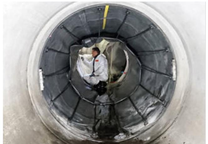
In contrast to „mobile solutions“, such as the installation of a pneumatically operated Sewer Sealing Cushions or a conventional pipe plug, the sewer shut-off system KAS offers the advantage that it does not lead to any conflict regarding valid working condition acts and a quick deployment, as neither the pipeline nor the manhole must be entered for the activation:
